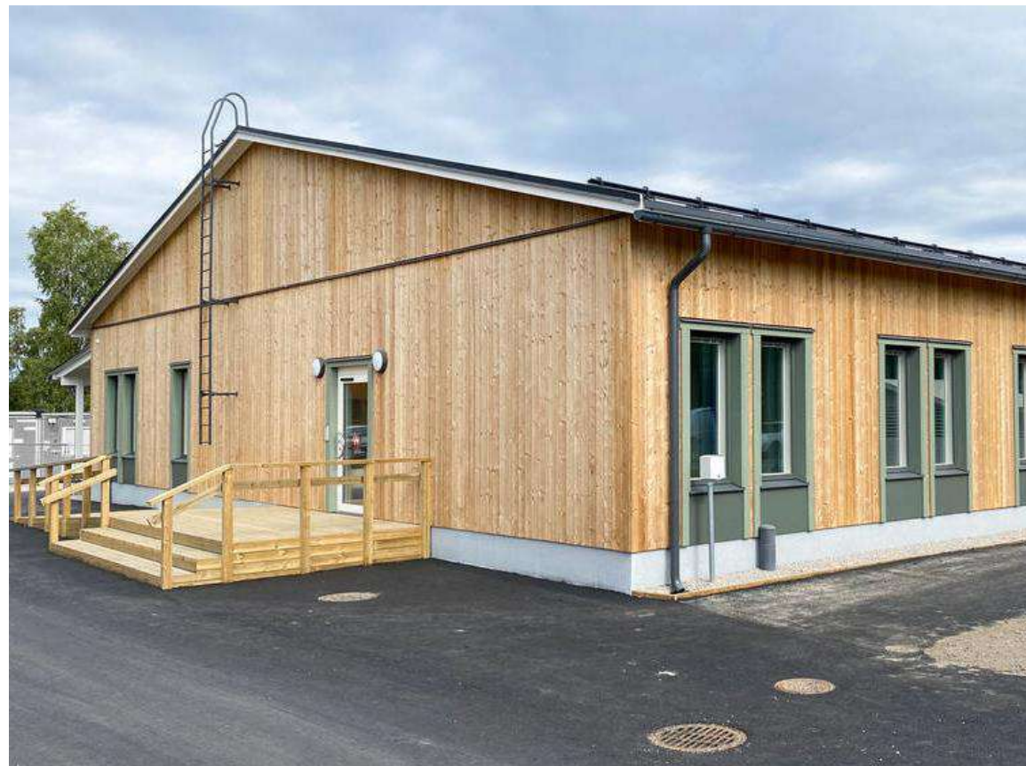
Service Center Kaskinen, Finland
